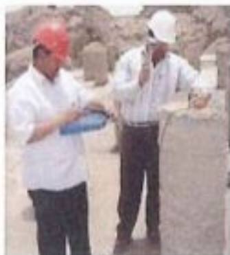
Fig.4 Test in progress
