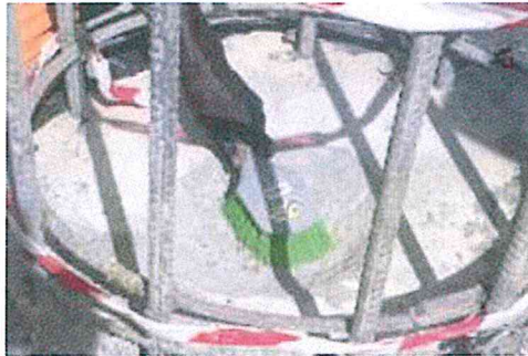
Fig.2 Pile head preparation
