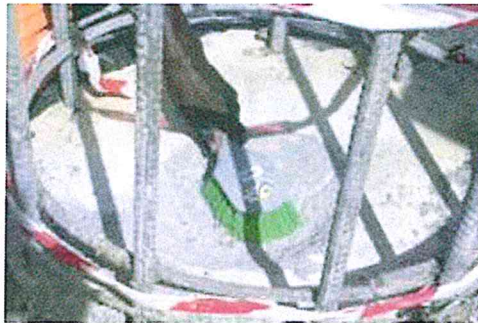
Fig.2 Pile head preparation
