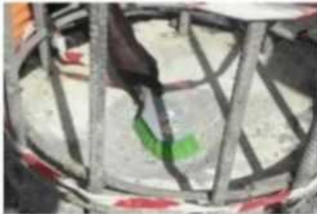
Fig.2 Pile head preparation
