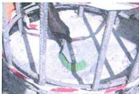
Fig.2 Pile head preparation
