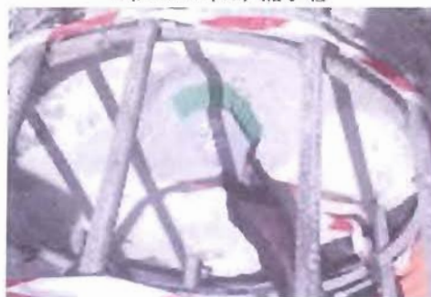
Fig.2 Pile head preparation
