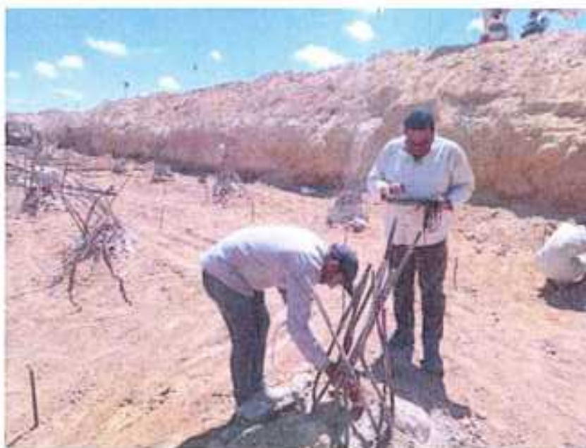
FIG. 1 SIT IN PROGRESS
